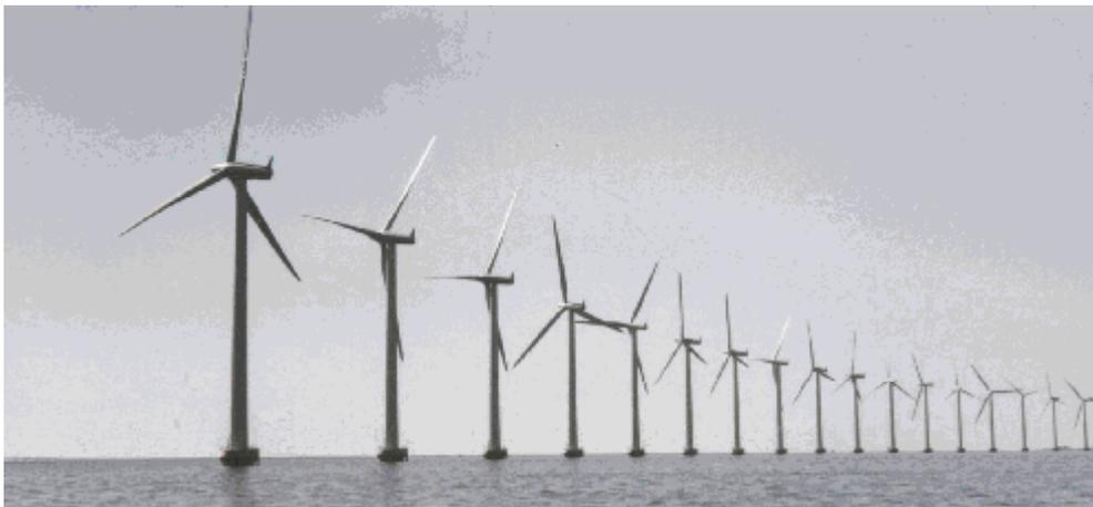
**Middelgrunden, a 40,000 KW wind farm offshore from Copenhagen, provides sufficient annual electricity for about 15,000 homes. Owned by a co-operative of 8,500 members, it has 20 turbines, with rotor diameters of 76 m.**
