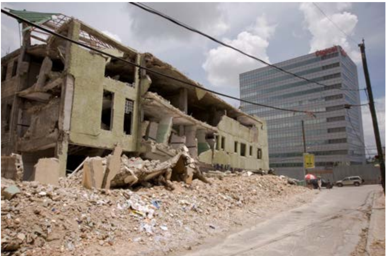
Comparison between response of two brand new buildings constructed in 2009 to the January 2010 earthquake in Haiti. Foreground is the collapsed 3-storey Turgeau hospital compared to background 13-storey Digicel phone company building where not a single window was cracked.
